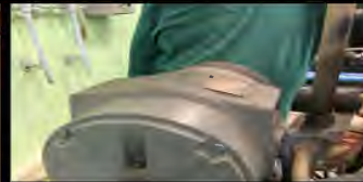
Pulled electric motor On #1 Air Compressor For Rebuild
