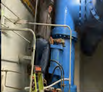
Started Dismantling #2 Backwash Pump for Rebuild
