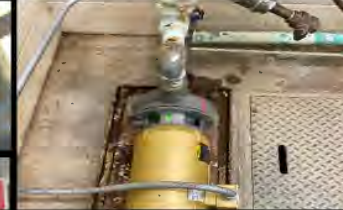
Installed New Screen Wash Pump
