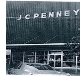
This building's architectural features have been totally obscured by a "modern" front. — 212 N. Penn, Independence, KS.
