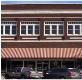
The "modern" front was removed from this building and the store front was restored. — 212 N. Penn, Independence, KS.
