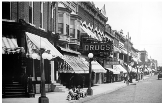
Try to locate old photographs or prints to determine what alterations have been made to the storefront and when they were undertaken. Awnings were common elements of storefronts at the turn of the century. — Northwest Corner of Penn/Main, Independence, KS.
